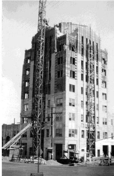
Hotel Baker opened in August 1929. Construction was completed in just 9 months.
